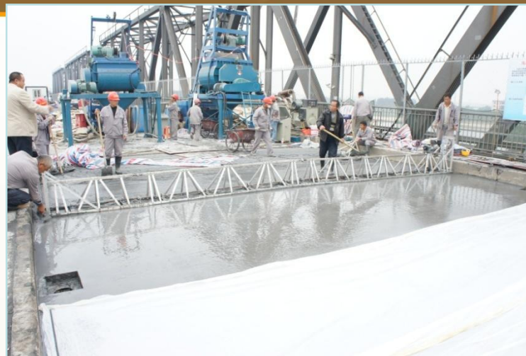
桥面现浇50mm厚STC层
